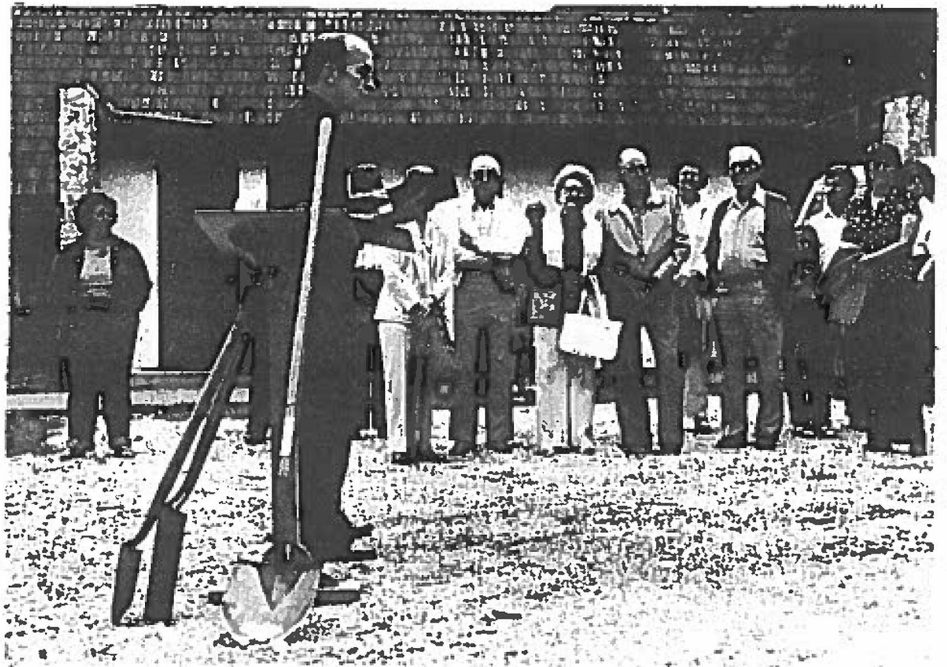
Ground Breaking on Labor Day
