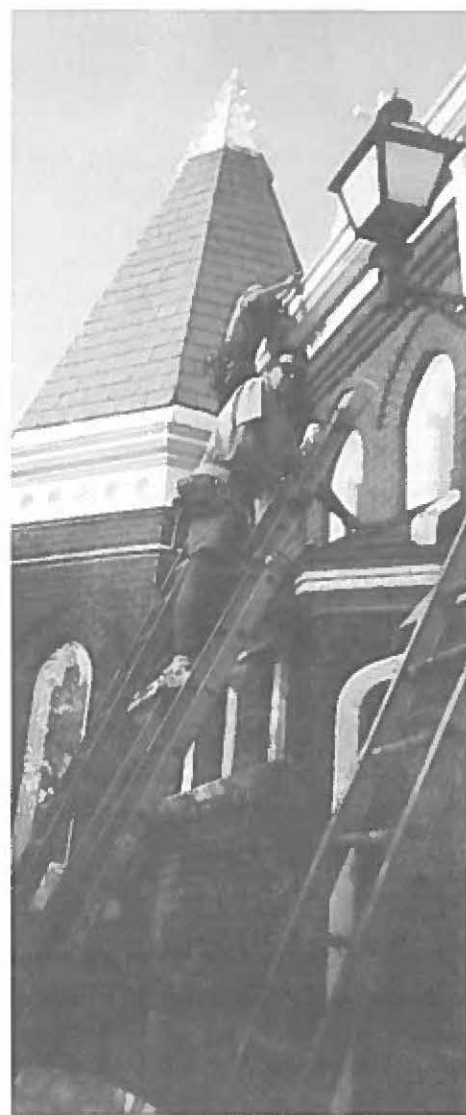
Work begins on the gutters, Monday, Aug. 12
