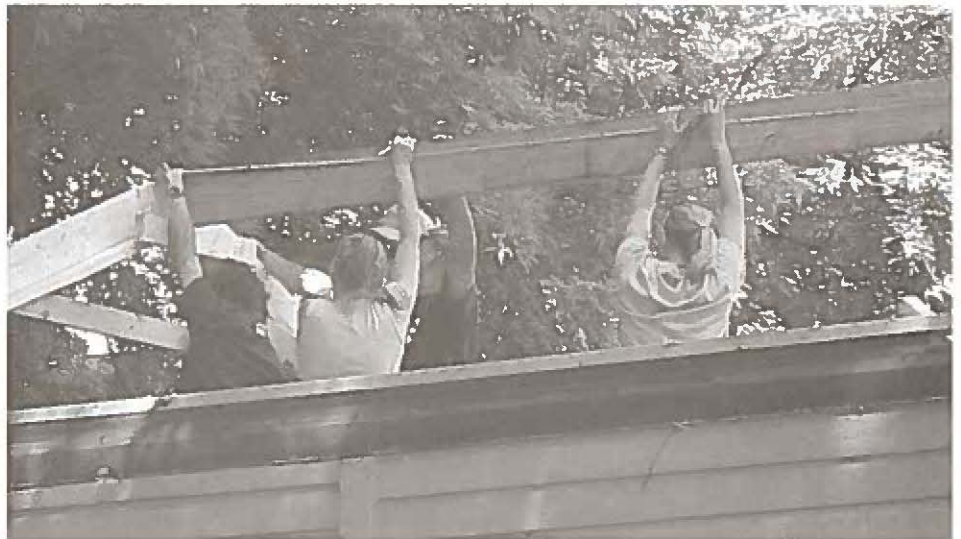
Setting the ridge board
