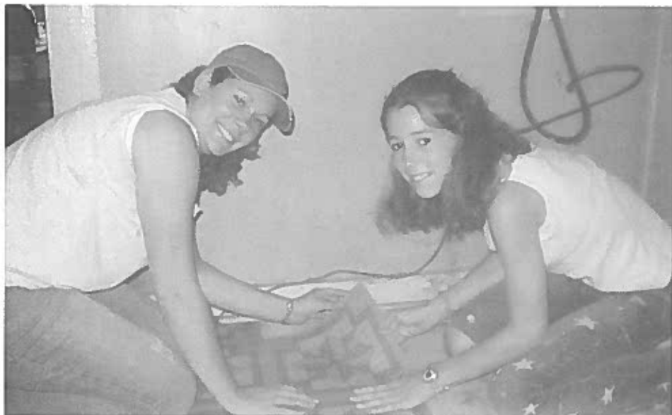
Laying a new floor was hard work, but we had fun doing it!
