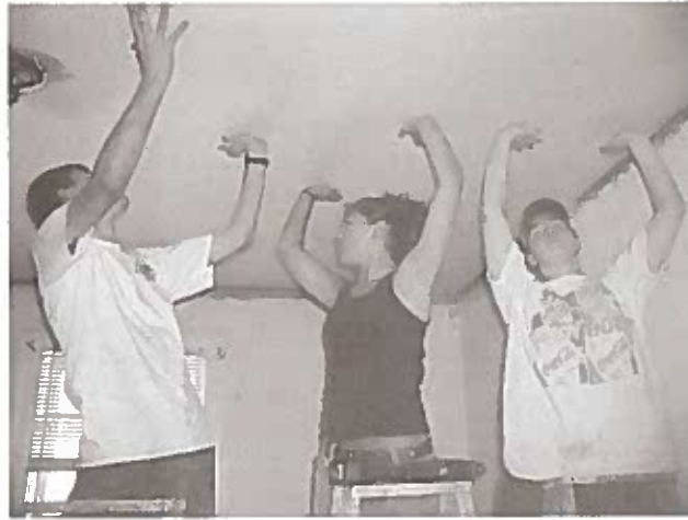
Working on the ceiling.
