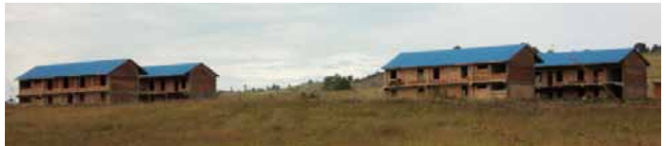
New buildings, in a lonely landscape, await a sewage system, bathrooms, window glass, and a fence to protect the school children from marauding animals.
