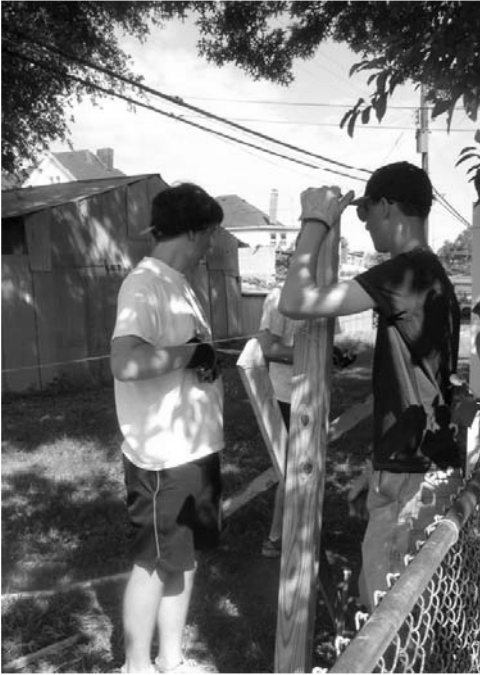
Chris and Kyle work on plumbing the new fence posts.
