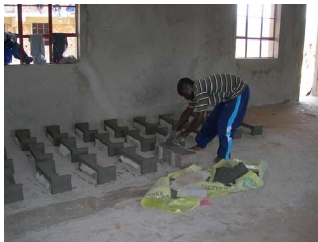
Preparing seating for one of the classrooms at Kwauso School
